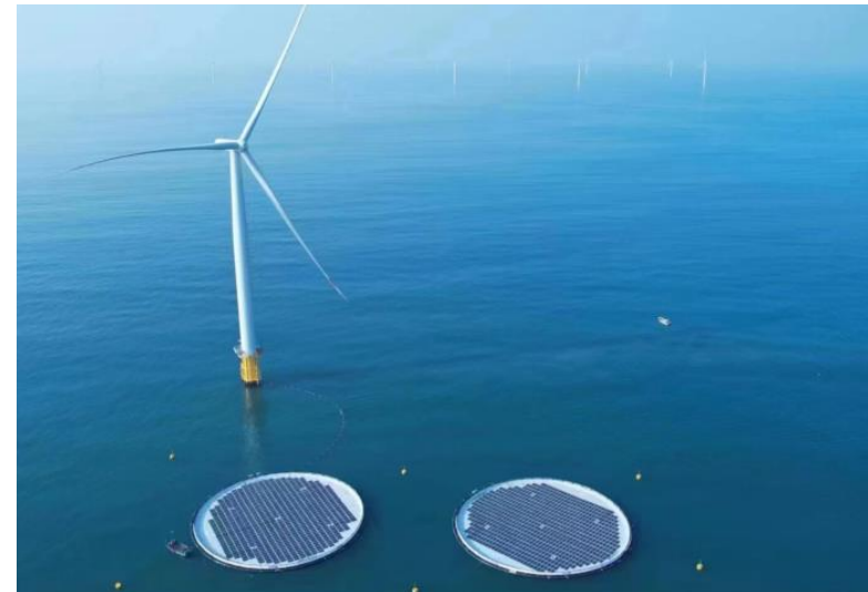
Floating PV system sharing infrastructure with offshore wind turbine. (Bernadette Geyer, June 26, 2023. Retrieved from: www.pv-magazine.com/2023/06/26/offshore-floating-vs-land-based-pv-systems/ )
